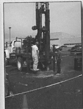
Drilling on Flat Terrain
