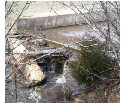
Lake Adams Outlet Structure
