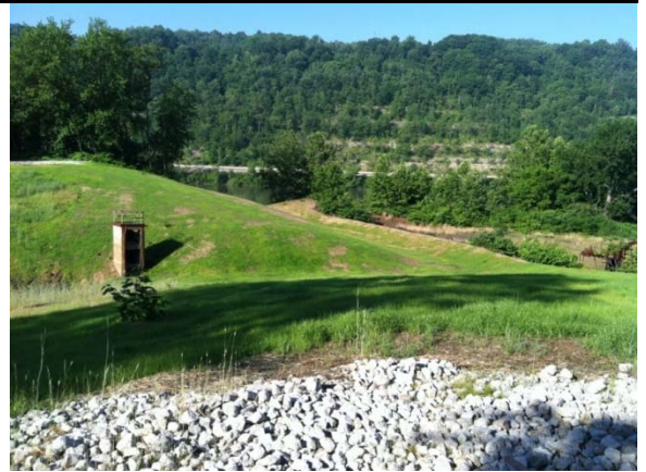
Drainage Channel at R.E. Burger Site
