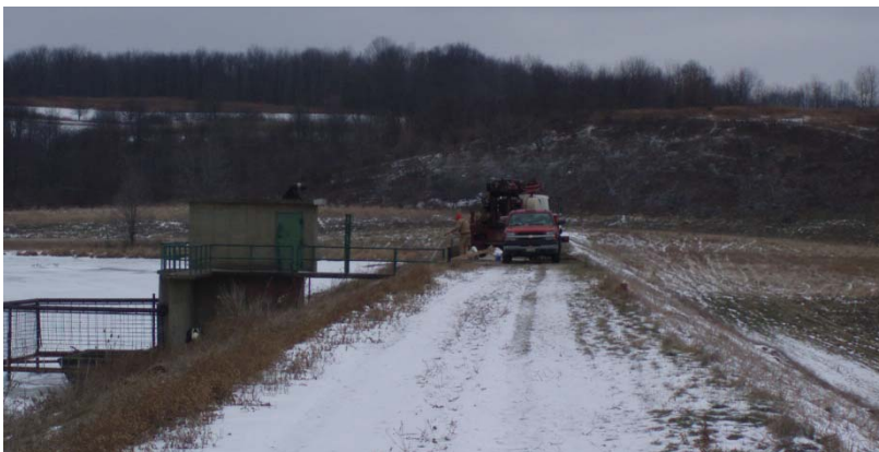
Geotechnical Investigation at Principal Spillway Structure
