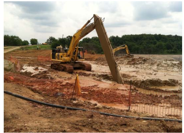
Slurry wall Construction at Little Blue Run Site
