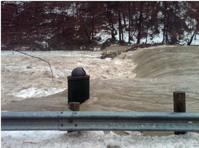
Gates Mill Dam Breach
