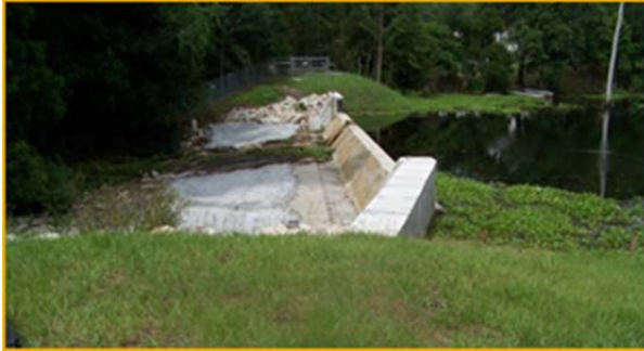
Completed dam in 2007
