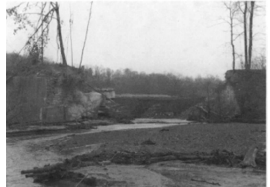
Ivex Dam Failure
