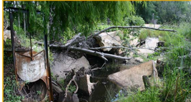
Damaged dam in 2005
