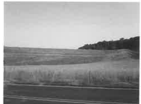
Embankment downstream slope and auxiliary spillway at Stony Creek #10 Dam
