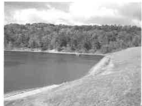
The upstream slope of the Stony Creek #9 Dam.
