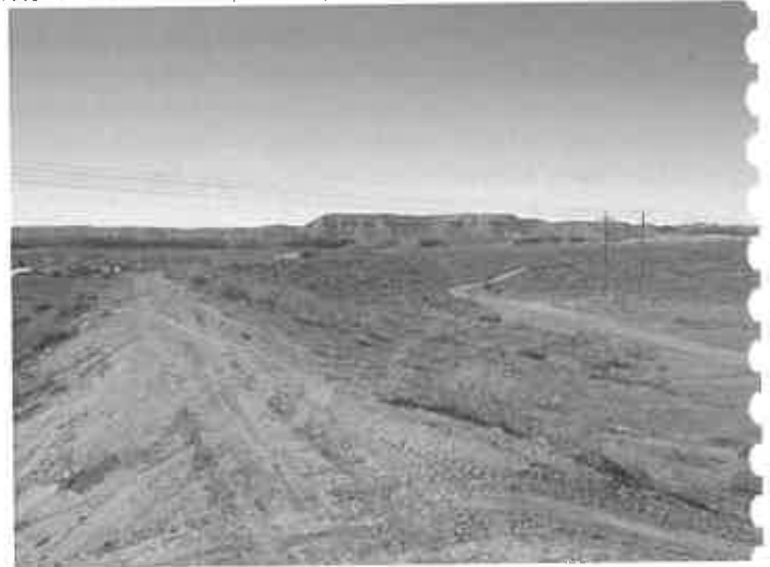
Fredonia FRS. Our team provided support for geotechnical design and construction reports on filter design, foundation soils, borrow material, and regional geology.
