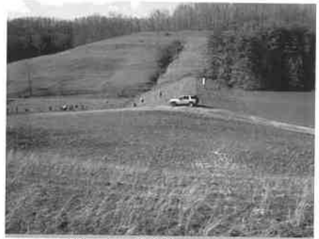
Salem Fork Site 11A. Gannett Fleming evaluated several spillway rehabilitation alternatives to comply with Class C high hazard design criteria and recommended armoring the auxiliary spillway.
