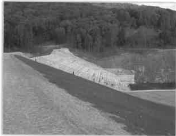
Figure 14: New Creek Site 14 Dam, WV. Gannett Fleming performed planning, analysis, design construction drawings, and specifications, permitting, and construction management on a fast-track schedule for this NRCS WV dam.
