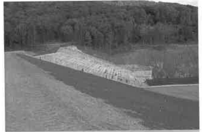
RCC Spillway at New Creek Site 14 Dam. Fly ash, a byproduct of coal-fired power generation, was used to replace 50 percent of the cement in all RCC used for this project. Using recycled materials resulted in significant energy and pollution savings by decreasing the Portland cement usage on this project by approximately 2,850 tons which results in CO 2 emissions and eliminates the need to landfill these industry by-products.
