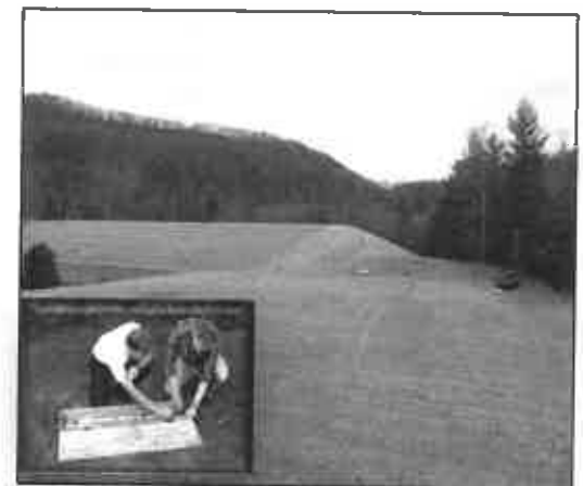
Figure 5: Lake Laura Dam. Our geologists and geotechnical engineers performed subsurface exploration and mapped the geologic profile of the auxiliary spillway at Lake Laura Dam to develop the erodibility parameters needed to evaluate the stability and integrity of the auxiliary spillways.
