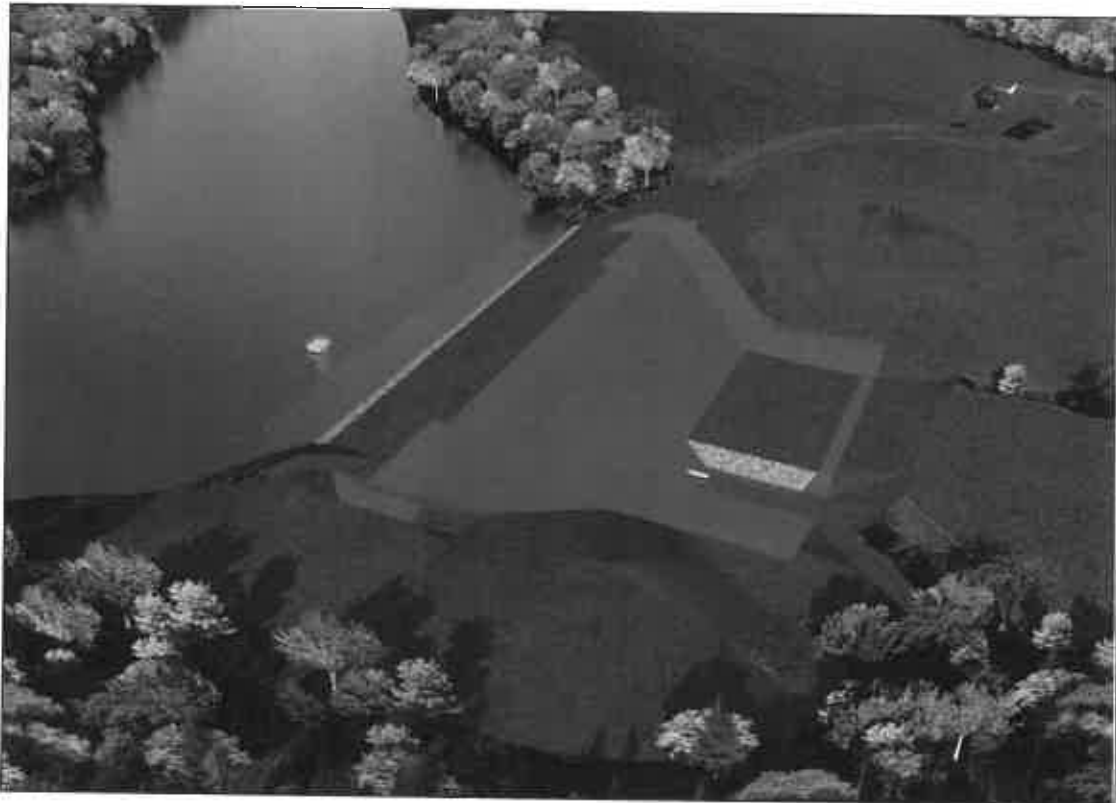
Figure 22: Upper Deckers Creek Site 1 Dam Rehabilitation. In this artist rendering of proposed modifications to Upper Decker's Site 1, RCC armoring is shown without vegetated soil cover to illustrate the extent of RCC armoring.
