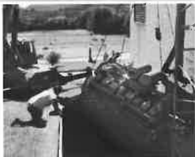
Crane lowering the emergency power generator into the electrical room.
