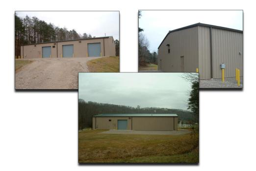
Prior to founding Three Designs, Mr. Bolen provided complete project architectural design services through bidding for a new pre-engineered metal building facility. The building was designed with a drive through bay, and two drive-in bays to the building. The site of the facility is located in Coonskin Park in Charleston, West Virginia.
