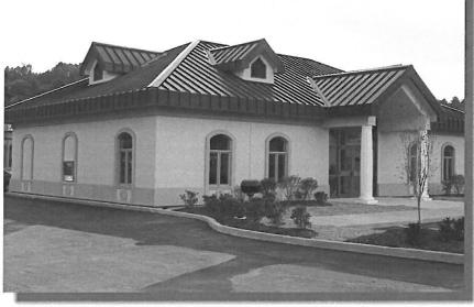
The Pioneer Community Bank is a new branch facility located at the Lester Square Shopping Center. The facility is constructed with wood frame, EIFS exterior, metal roof, aluminum entry and clad windows providing a maintenance free exterior.
