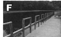
Illustration of a typical ADA Fishing Pier. The relocation of the ADA Fishing Pier allows for easier access and better circulation at Bee Run Marina.
