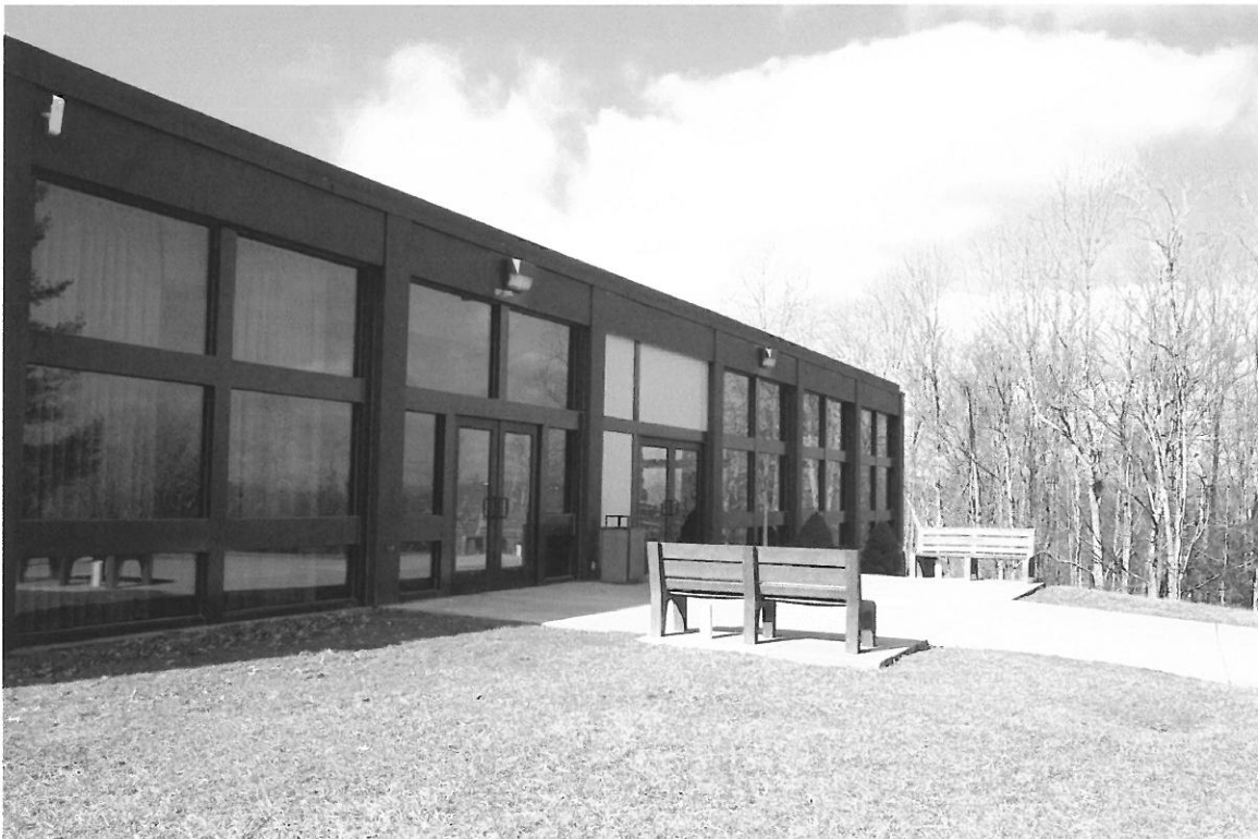
Pipestem Conference Center Addition
