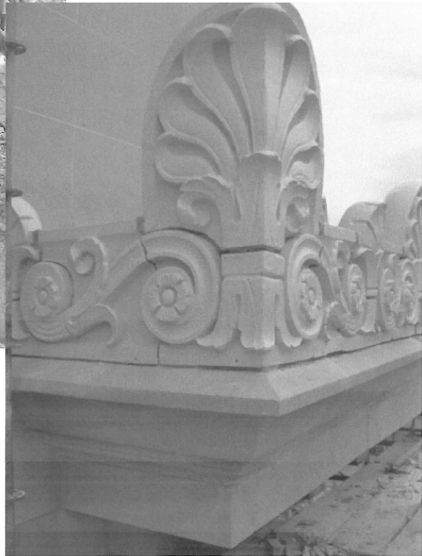
Portions of the limestone cornice were damaged to the point that they fell when work was being conducted and had to be pinned back in place.
