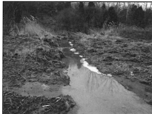
Site before remediation showing poor vegetation and water quality, rills and gullies
