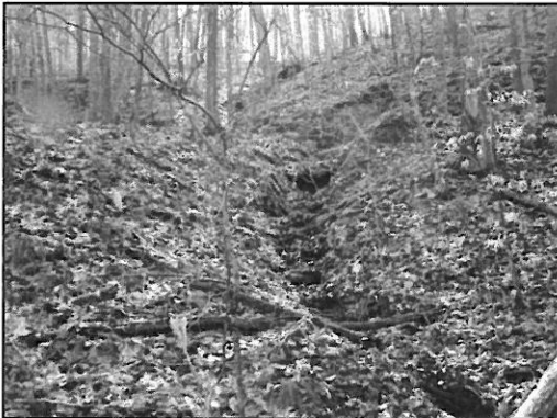
Eroded drainage path from bench
