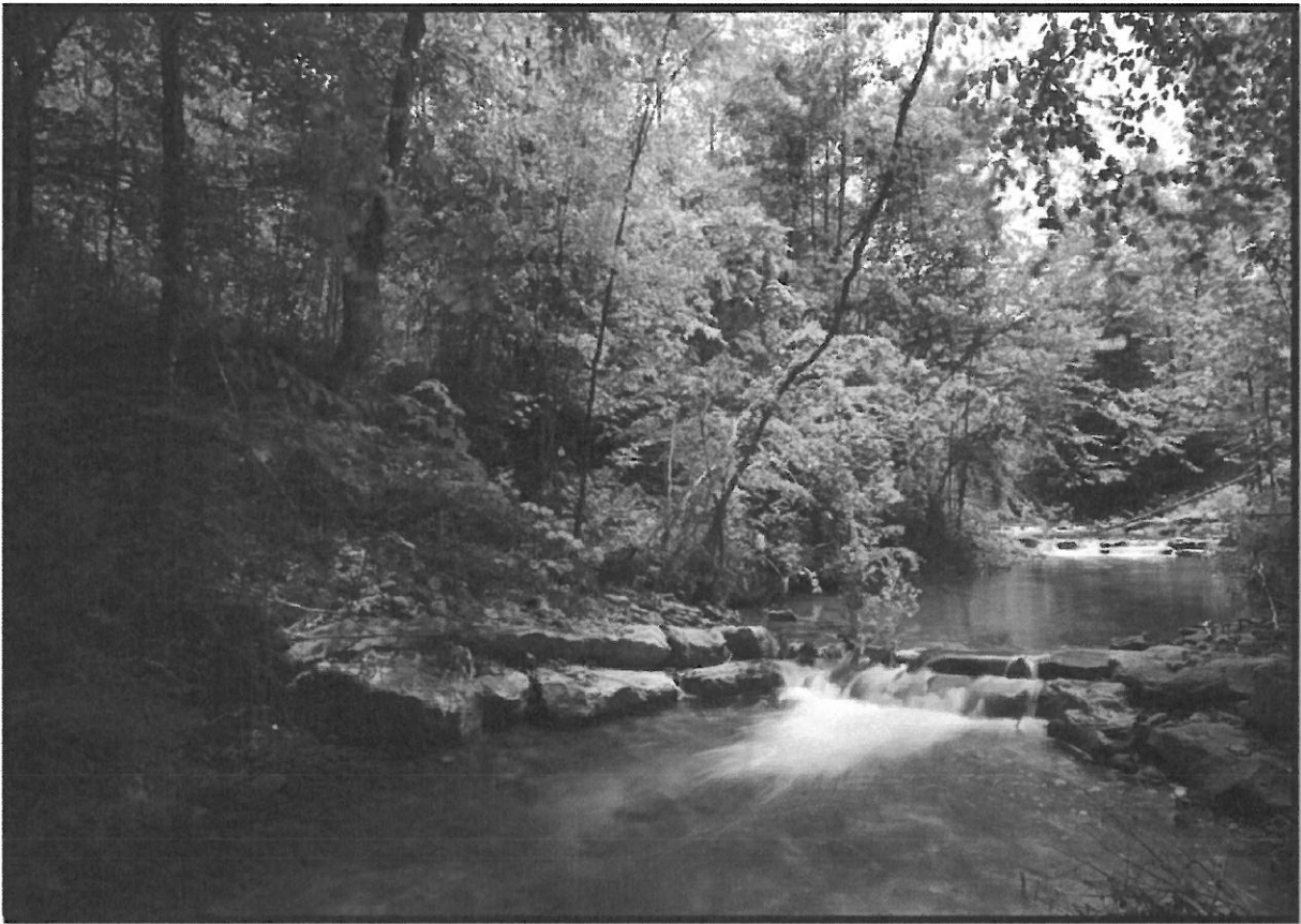
Rock cross vane- one of a series of structures used to stabilize a section of stream which had been realigned.
