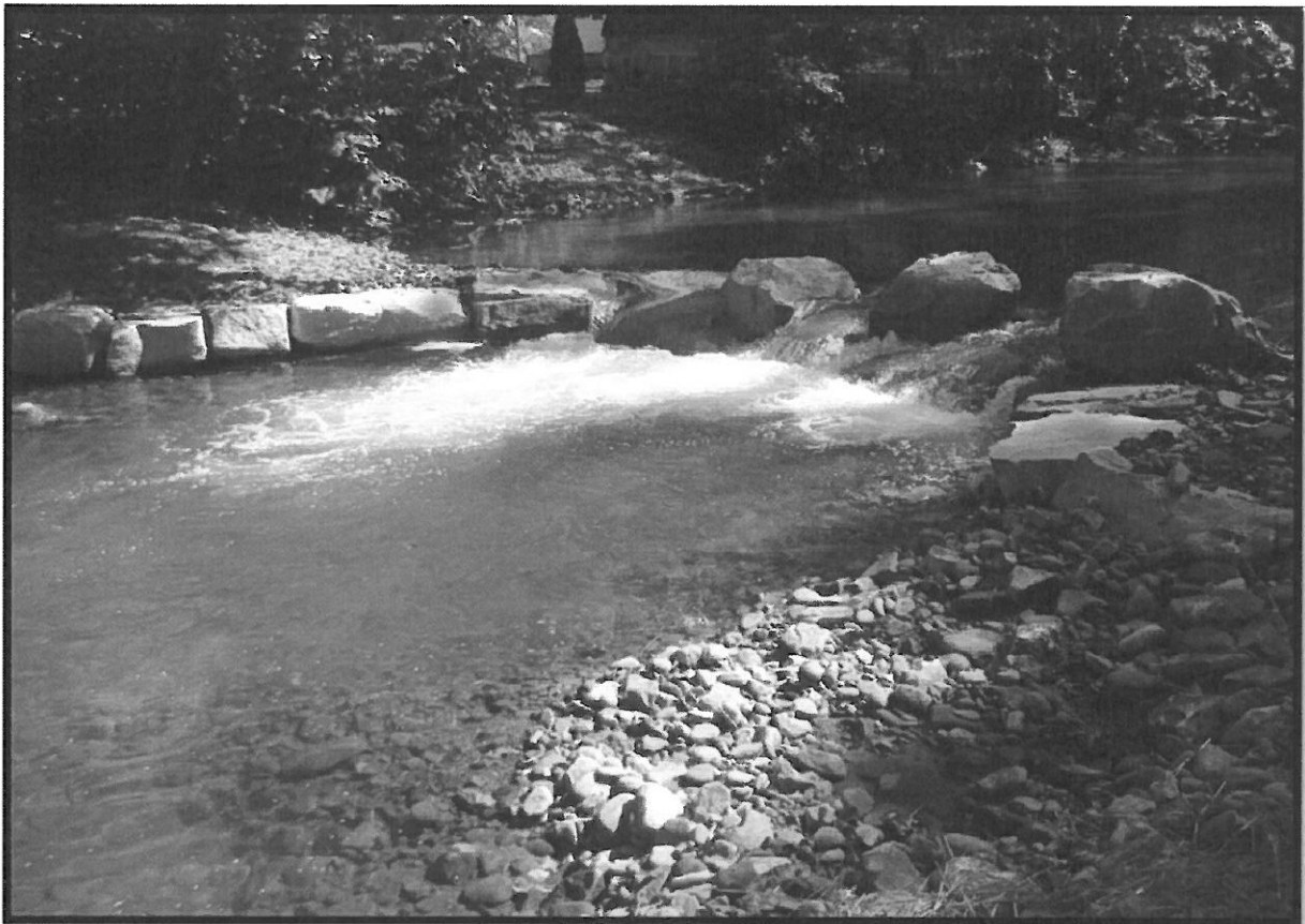
J-hook structure on Paint Creek
