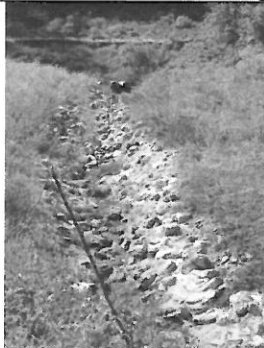
NIXON RUN AMD: Wet Mine Seal outlet pipes and receiving ditch.
