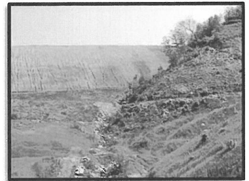
Downstream - Post Stage III Construction
