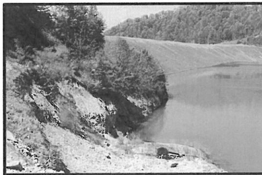
Upstream - Post Stage III Construction
