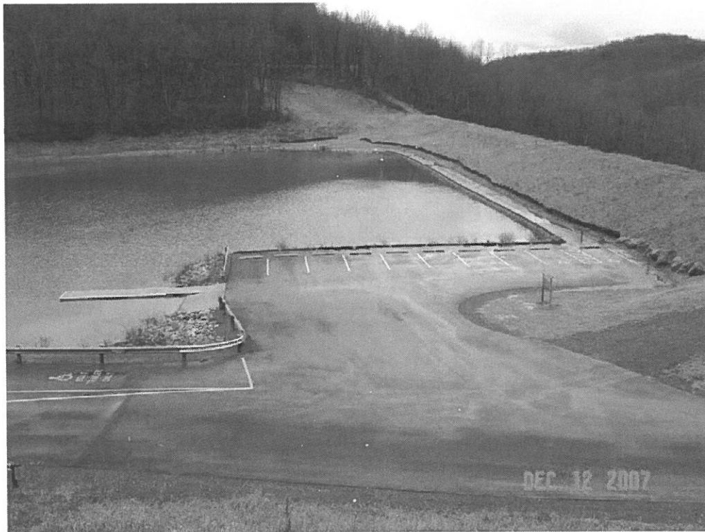
BAILEY DAM MODIFICATION, MONONGALIA CO., WV
