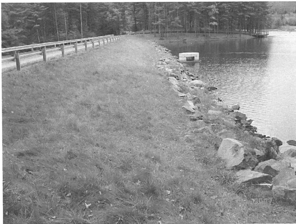
MONCOVE DAM MODIFICATION, MONROE CO., WV
