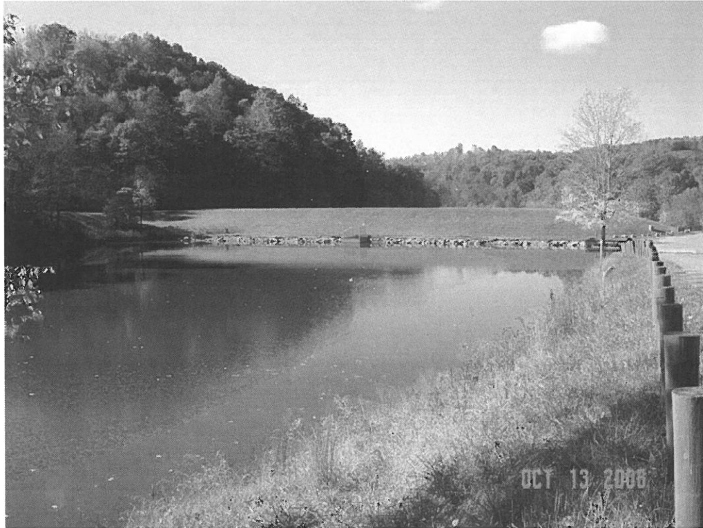
JIMMY LEWIS DAM MODIFICATION, MERCER CO., WV
