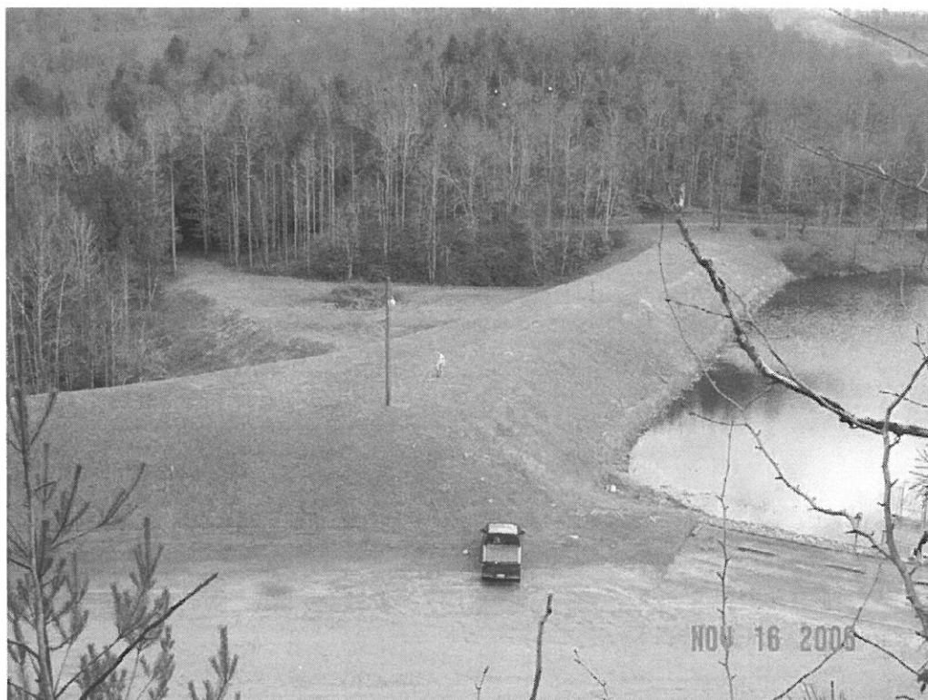
PLUM ORCHARD DAM MODIFICATION, FAYETTE CO., WV
