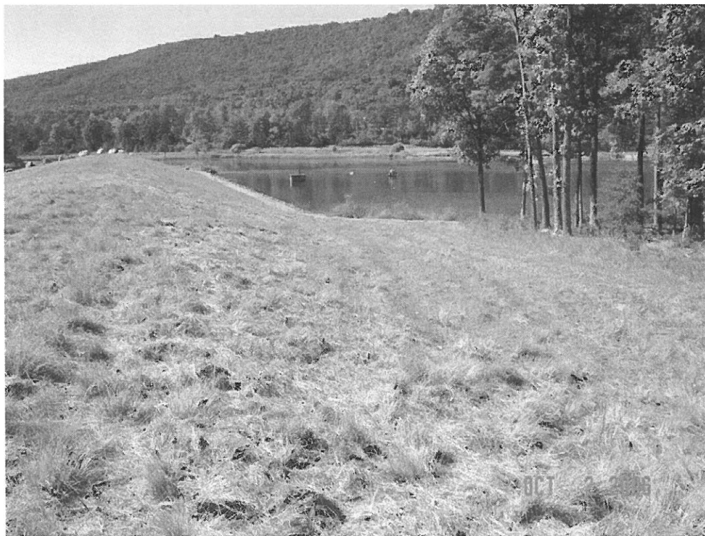
WARDEN LAKE DAM MODIFICATION, HARDY CO., WV
