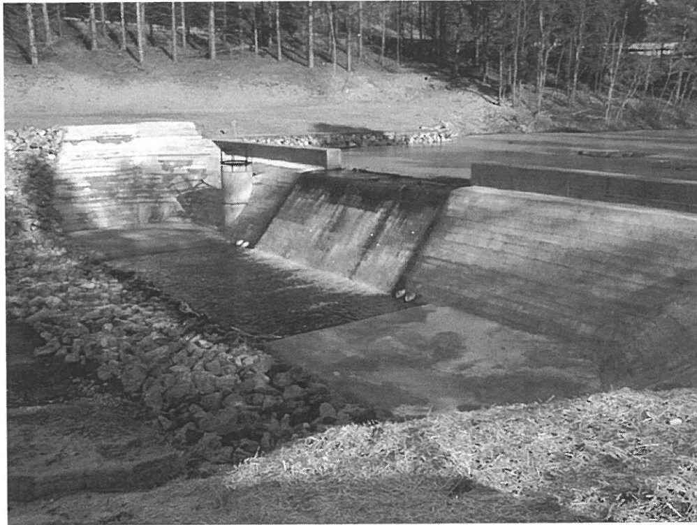
THOMAS DAM MODIFICATION, THOMAS, WV
