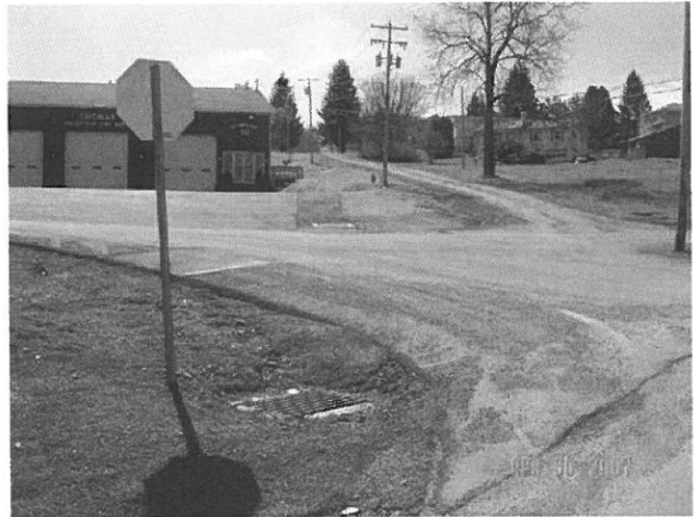
New Storm Drains and Catch Basins
