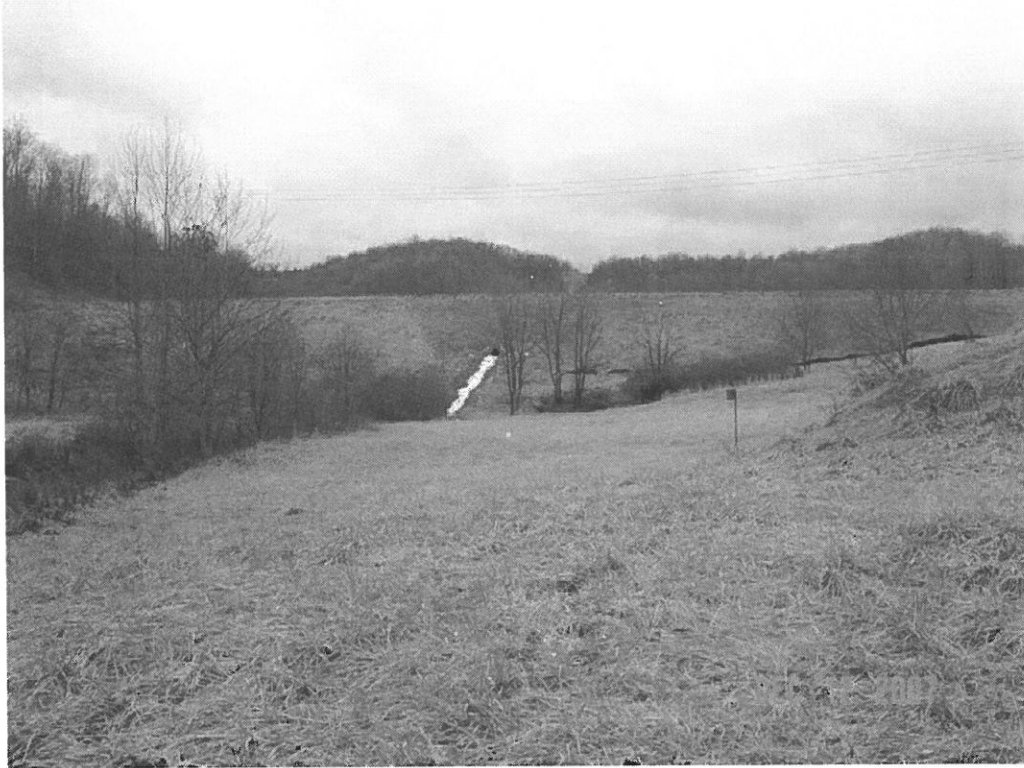
LEMLEY DAM MODIFICATION, MONONGALIA CO., WV
