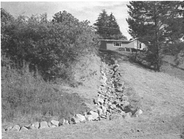
Erosion Repair – Rip Rap Armored Ditch
