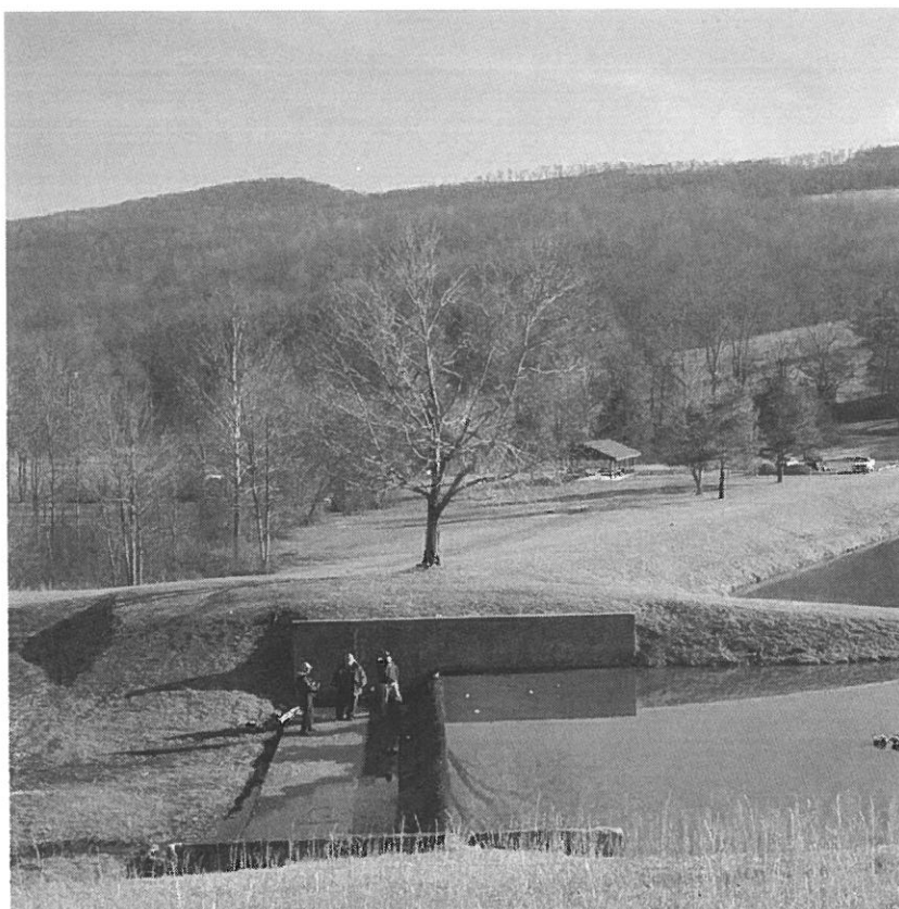
BELINGTON DAM MODIFICATION, BELINGTON, WV
