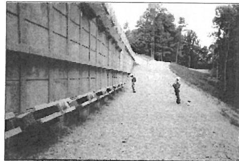
Finished wall with anchors
