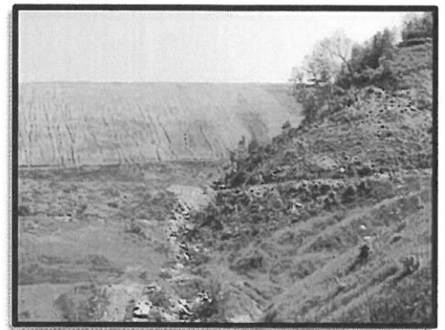
Downstream - Post Stage III Construction
