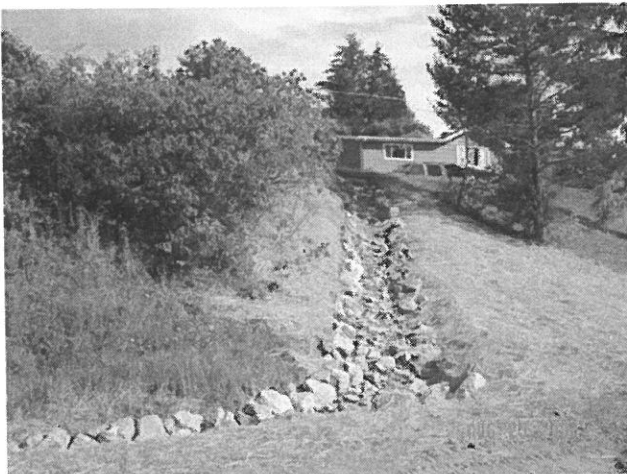
Erosion Repair – Rip Rap Armored Ditch
