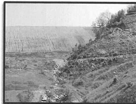
Downstream - Post Stage III Construction
