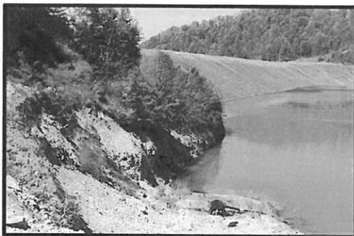
Upstream - Post Stage III Construction
