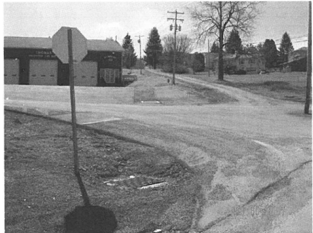
New Storm Drains and Catch Basins
