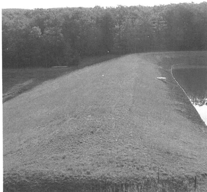
WILSON DAM MODIFICATION, HAMPSHIRE CO., WV
