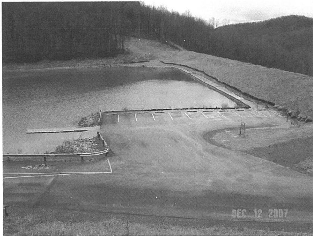
BAILEY DAM MODIFICATION, MONONGALIA CO., WV
