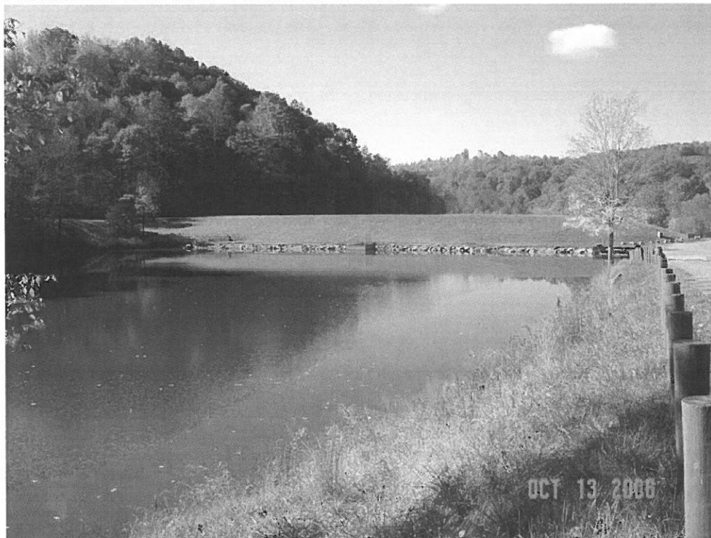
JIMMY LEWIS DAM MODIFICATION, MERCER CO., WV
