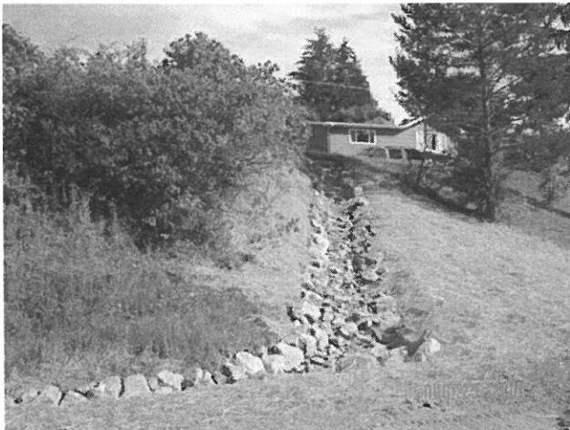
Erosion Repair – Rip Rap Armored Ditch
