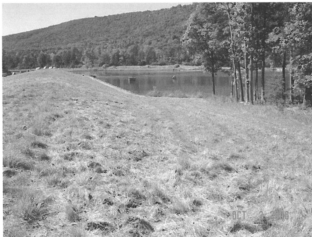
WARDEN LAKE DAM MODIFICATION, HARDY CO., WV
