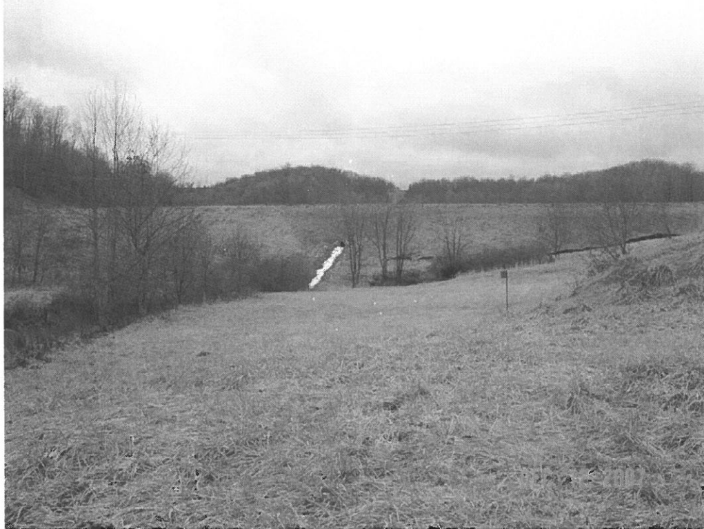
LEMLEY DAM MODIFICATION, MONONGALIA CO., WV
