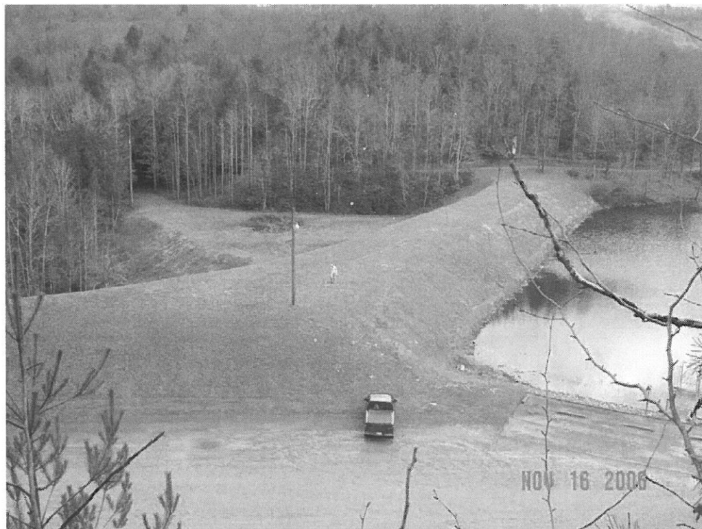
PLUM ORCHARD DAM MODIFICATION, FAYETTE CO., WV
