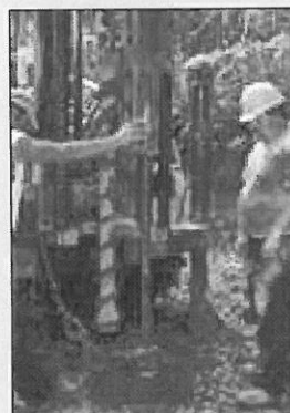
Drilling in Rugged Terrain
