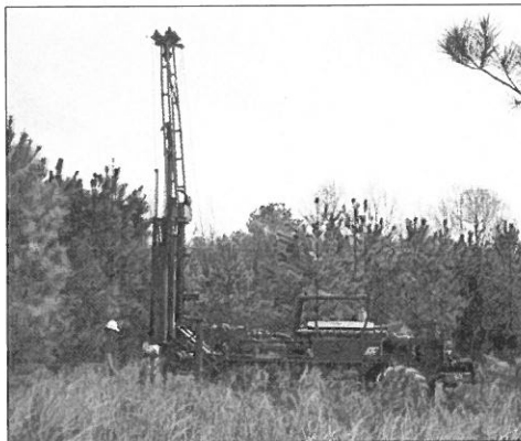
CTL's ATV can drill in rough terrain
