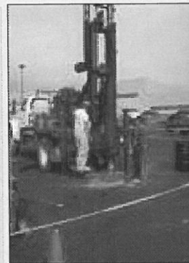
Drilling on Flat Terrain
