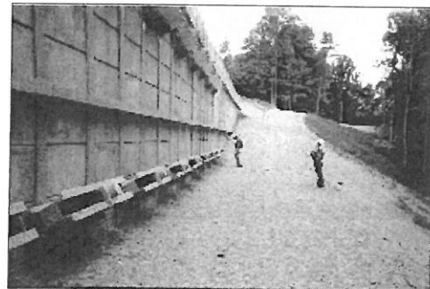
Finished wall with anchors
