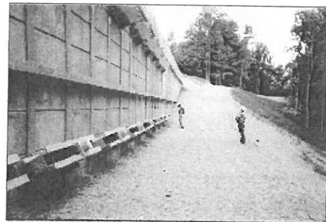
Finished wall with anchors
