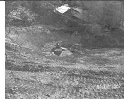
PRICE HILL AIRSHAFT AND BUILDINGS: Vertical mine shaft sealing in progress.
