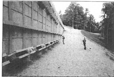
Finished wall with anchors
