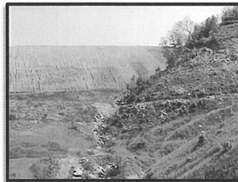
Downstream - Post Stage III Construction
