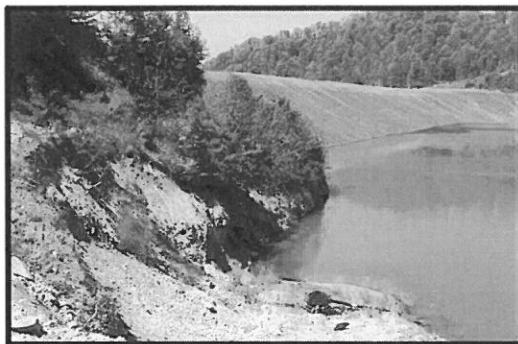
Upstream - Post Stage III Construction
