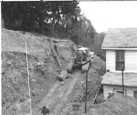
TUNNELTON (DILLSWORTH) LANDSLIDE Gabion Basket Wall Installation behind Dillsworth Residence
