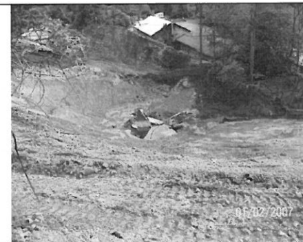
PRICE HILL AIRSHAFT AND BUILDINGS: Vertical mine shaft sealing in progress.
