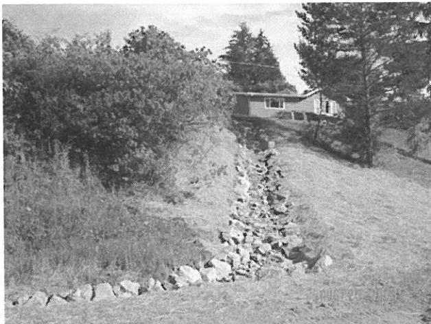
Erosion Repair – Rip Rap Armored Ditch
