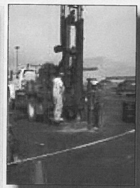
Drilling on Flat Terrain
