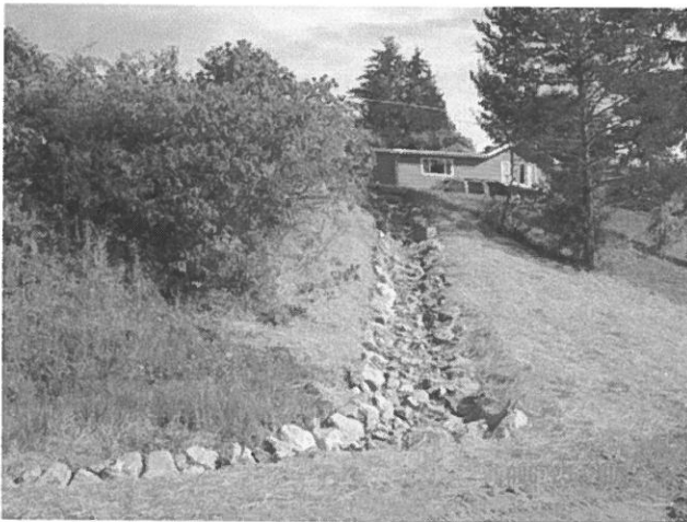
Erosion Repair – Rip Rap Armored Ditch
