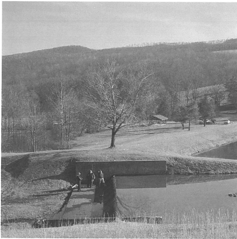
BELINGTON DAM MODIFICATION, BELINGTON, WV
