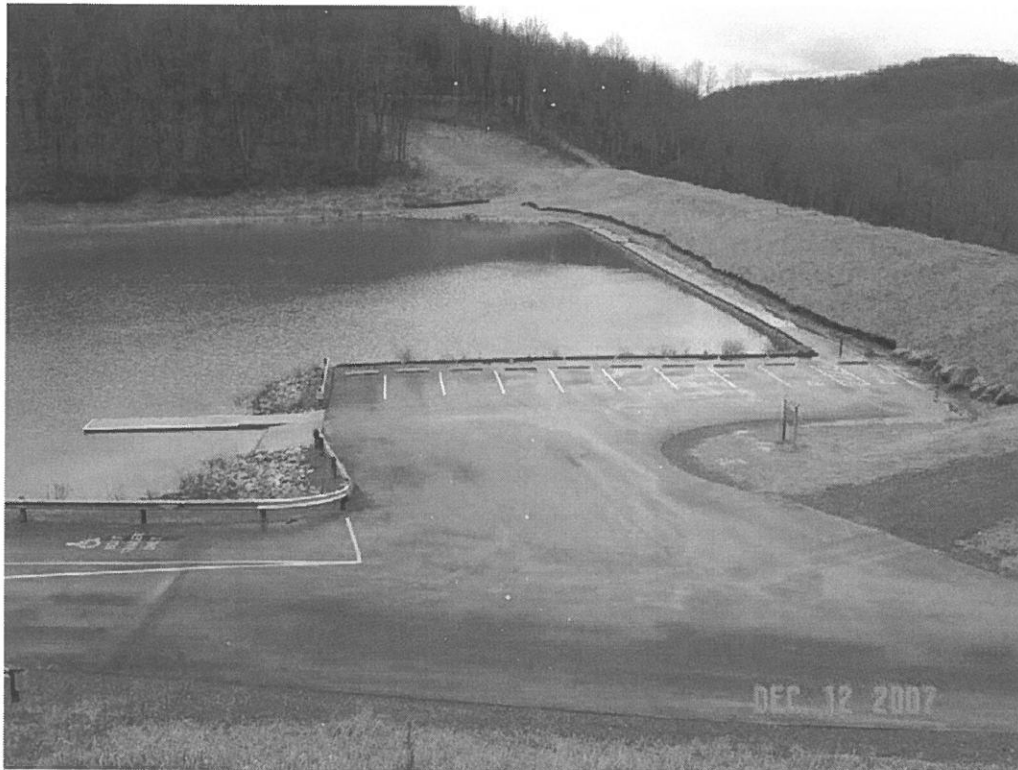
BAILEY DAM MODIFICATION, MONONGALIA CO., WV
