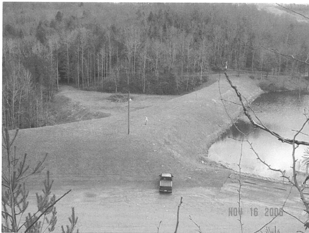
PLUM ORCHARD DAM MODIFICATION, FAYETTE CO., WV
