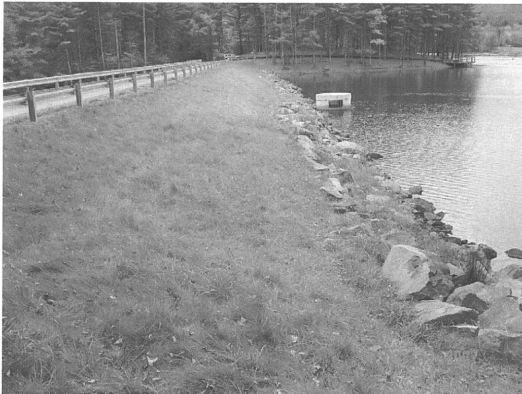
MONCOVE DAM MODIFICATION, MONROE CO., WV
