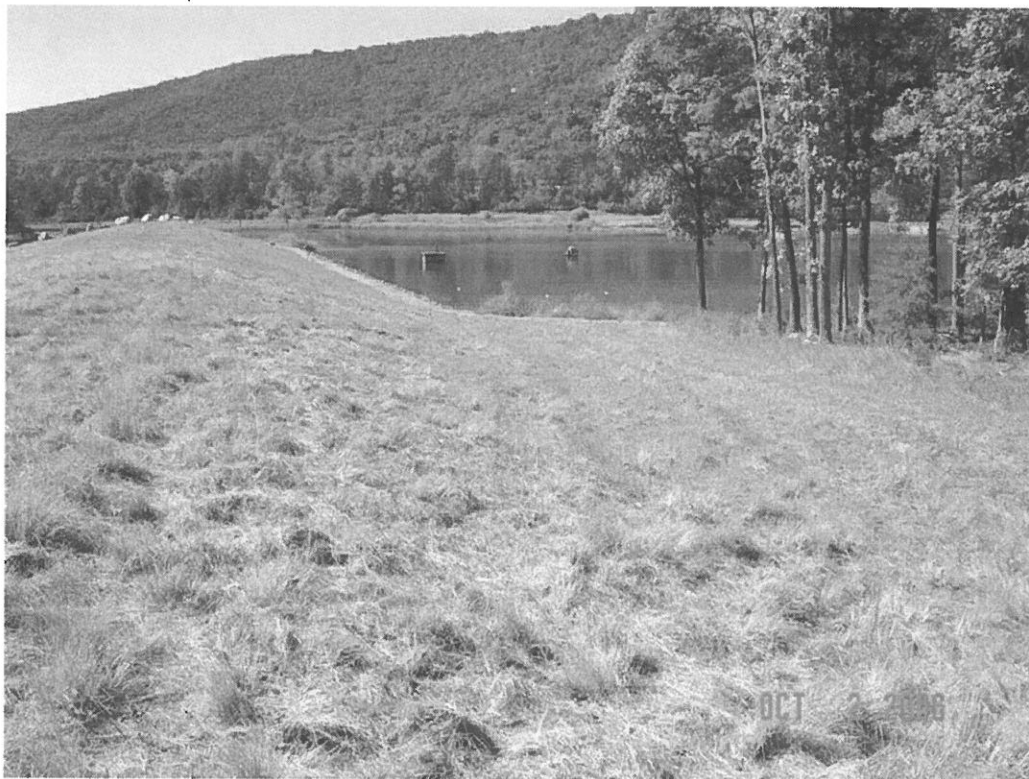
WARDEN LAKE DAM MODIFICATION, HARDY CO., WV
