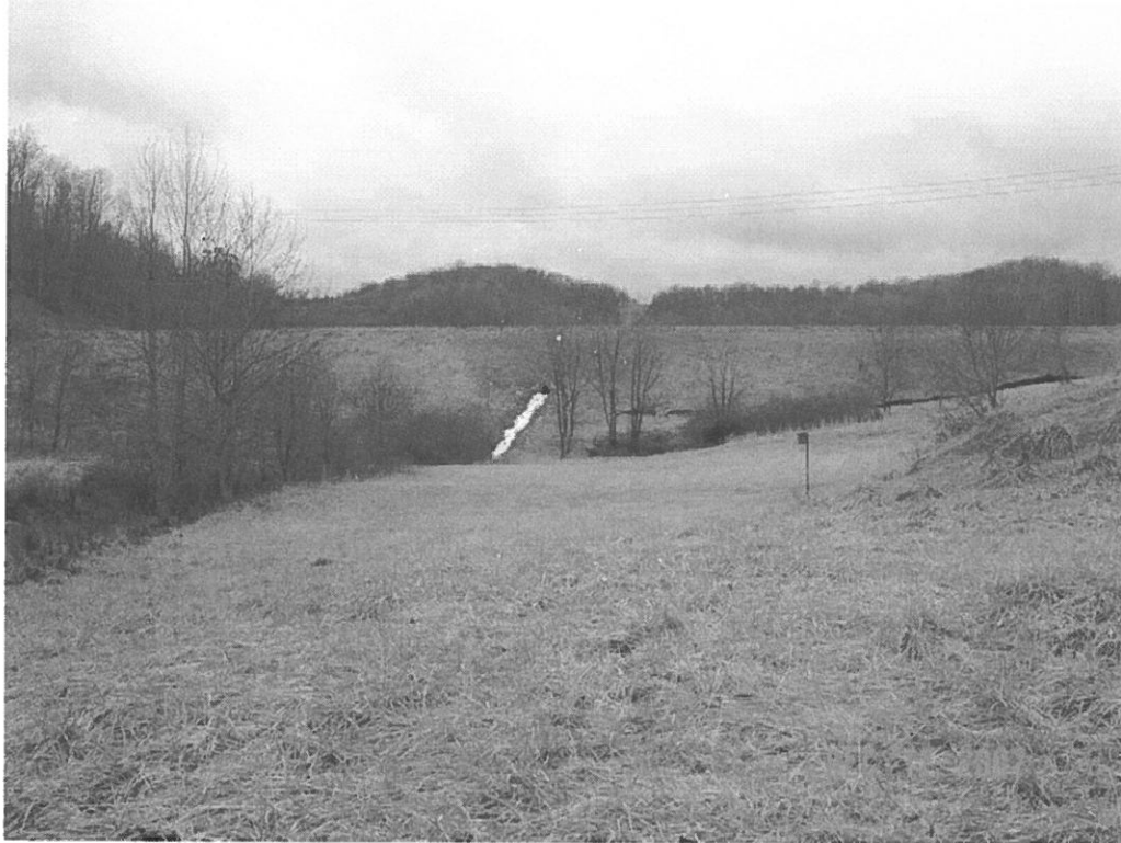
LEMLEY DAM MODIFICATION, MONONGALIA CO., WV
