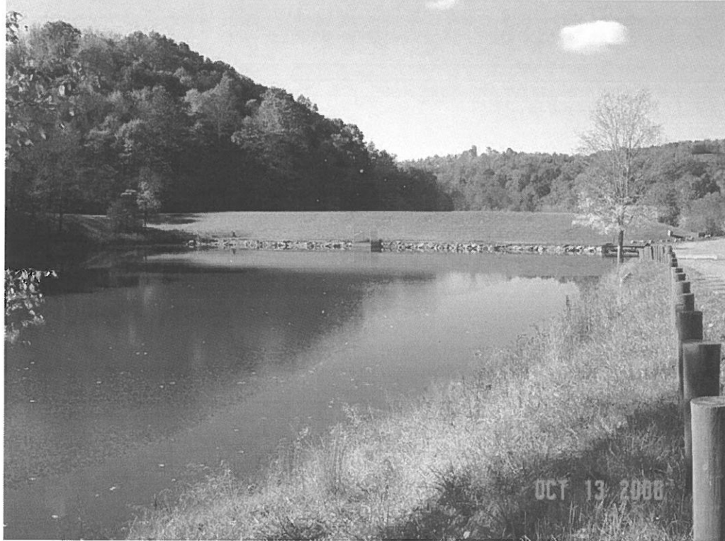
JIMMY LEWIS DAM MODIFICATION, MERCER CO., WV
