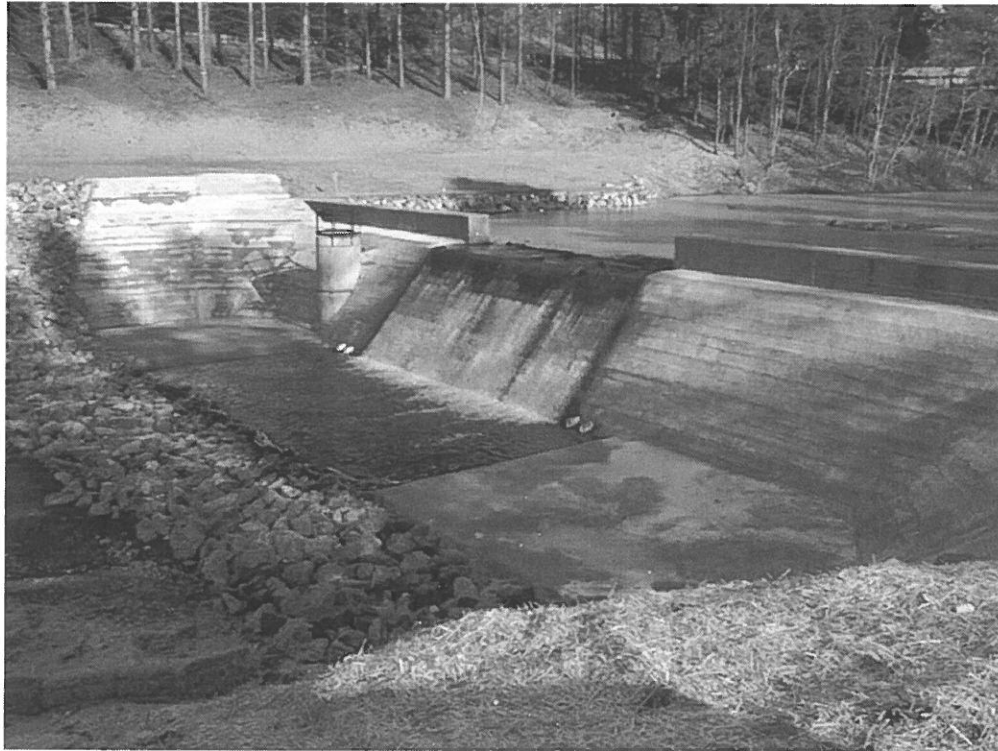
THOMAS DAM MODIFICATION, THOMAS, WV
