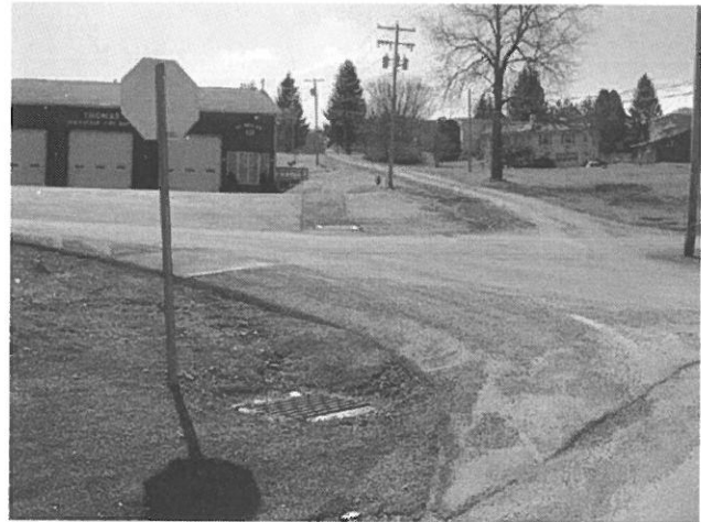
New Storm Drains and Catch Basins
