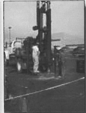
Drilling on Flat Terrain
