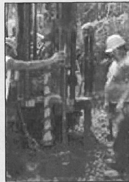
Drilling in Rugged Terrain
