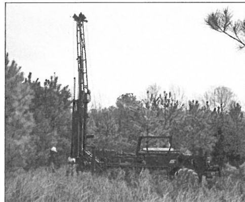
CTL's ATV can drill in rough terrain
