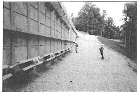
Finished wall with anchors
