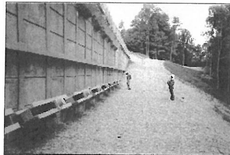
Finished wall with anchors
