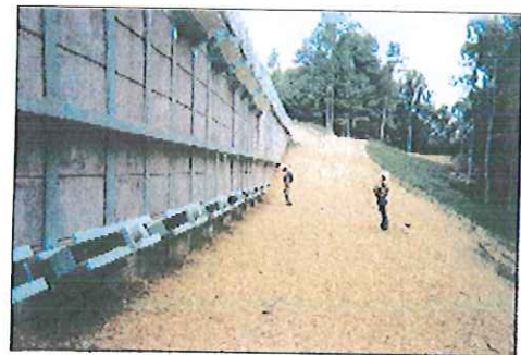
Finished wall with anchors
