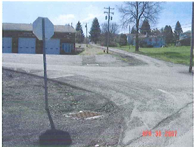
New Storm Drains and Catch Basins
