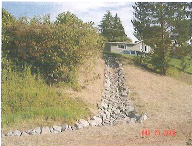
Erosion Repair – Rip Rap Armored Ditch
