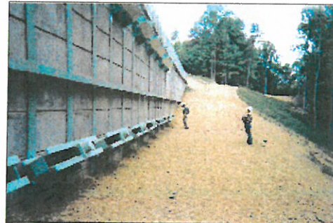
Finished wall with anchors
