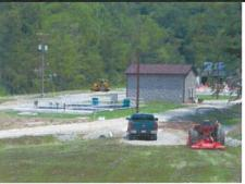
SPEC REC: Glady Fork Mining, Permit D-35-82 Bond Forfeiture alkaline mine drainage active chemical treatment facility. Along Stonecoal Creek near Buckhannon West Virginia.
