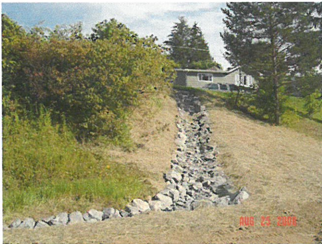
Erosion Repair – Rip Rap Armored Ditch
