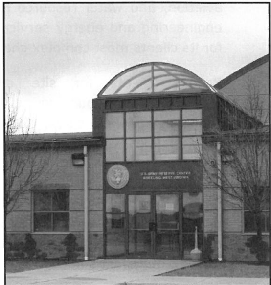
Design/Build of U.S. Army Reserve Training and Maintenance Center, Wheeling, WV
