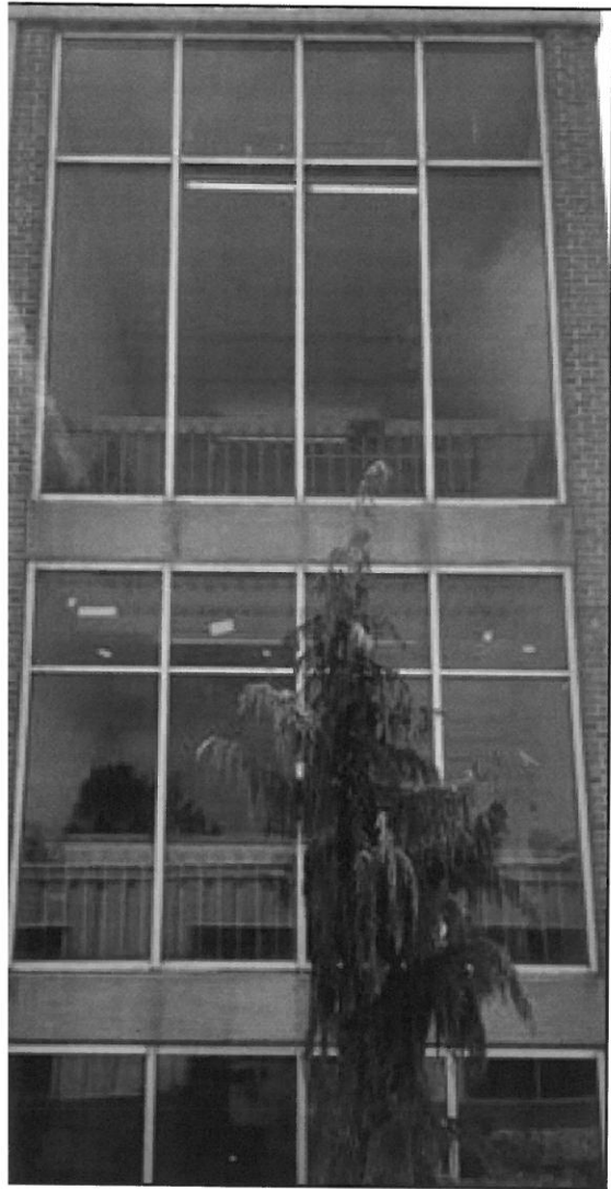
Mount View High School windows prior to replacement.
