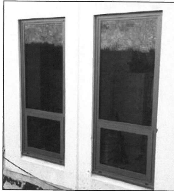
Mount View High School replacement windows are being installed.
