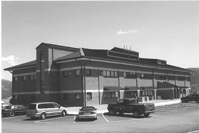
DISTRICT 6 OFFICE BLDG
