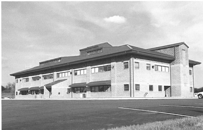
DISTRICT 10 OFFICE BLDG
