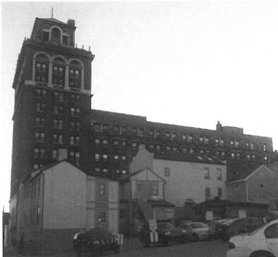
McKinley & Associates' Washington, PA Office
