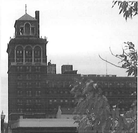
McKinley & Associates' Washington, PA Office
