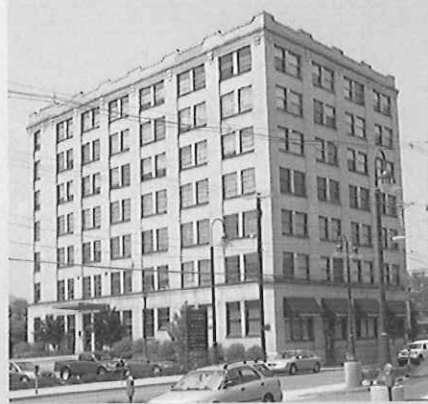
WAGNER BUILDING Wheeling, West Virginia
