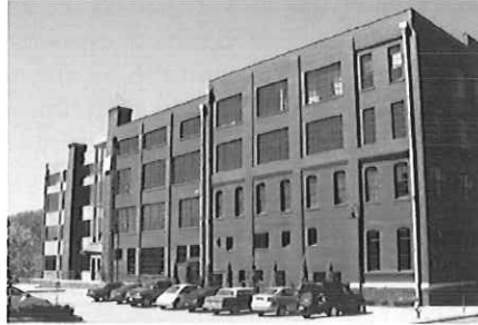
ORRICK BUILDING Wheeling, West Virginia
