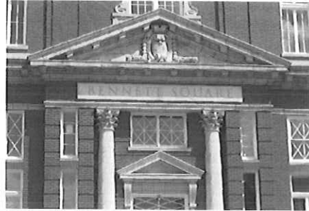
BENNETT SQUARE Wheeling, West Virginia
