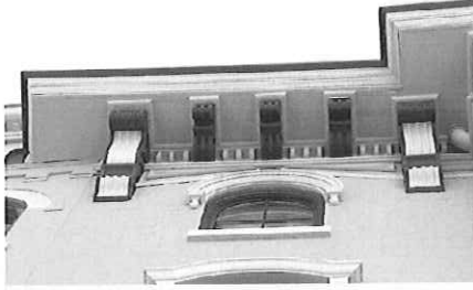
CATHOLIC HERITAGE CENTER Wheeling, West Virginia
