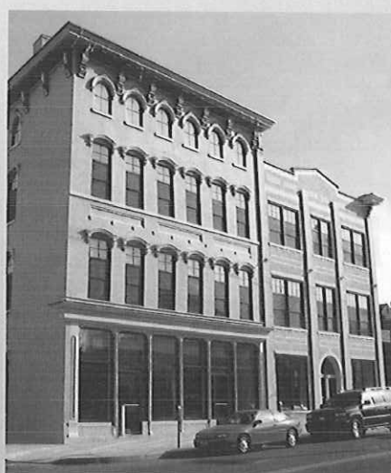
CATHOLIC HERITAGE CENTER Wheeling, West Virginia
