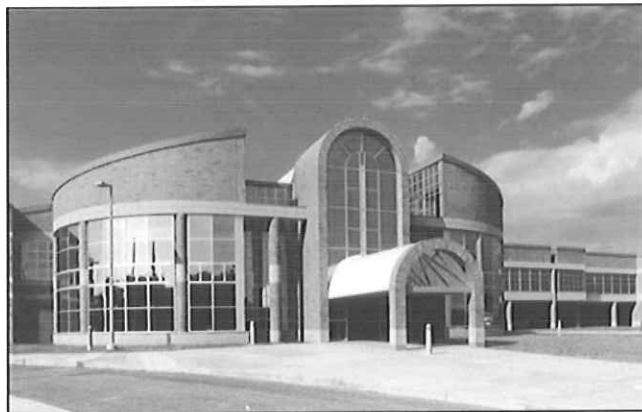
William R. Sharpe Jr. Hospital Weston, WV $30 Million
