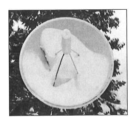
Repeated heavy snowfalls will stretch the panels of mesh and perforated dishes, reducing the accuracy of the reflective surface. Particularly heavy snowfalls will cause the panels to pop out of the channels, and can actually bend the mounts. The added weight of snow puts unnecessary stress on the actuator and motor, and can cause premature failure of either or both.
