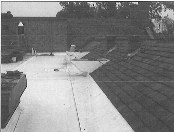
New Roof Construction - Final Completion
