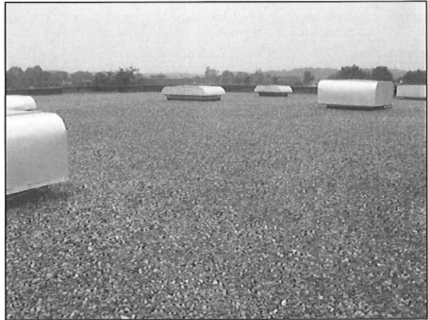
Roof Area Prior to Design by CTL
