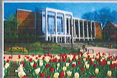
ZDS designed a system allowing West Virginia University to optimize their operation of the campus chilled water system.
