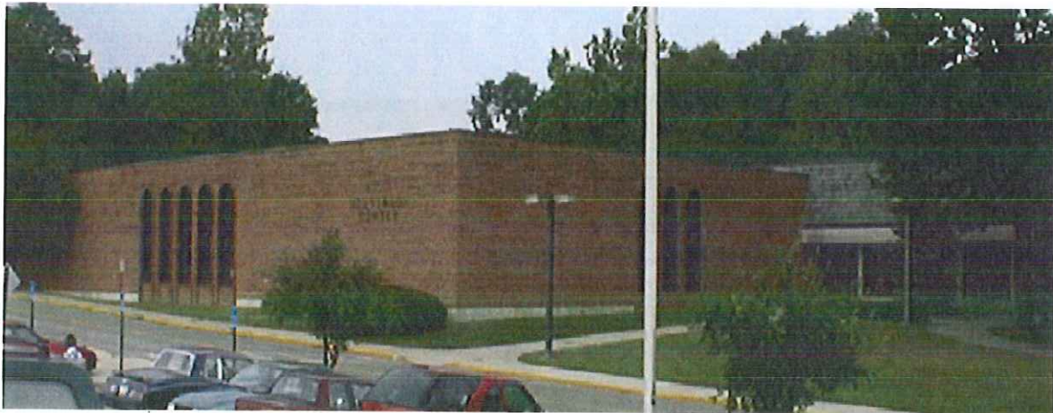
Stevenson Library – Renovations
