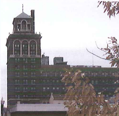
McKinley & Associates' Washington, PA Office
