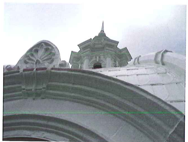
Dome Restoration Detail
