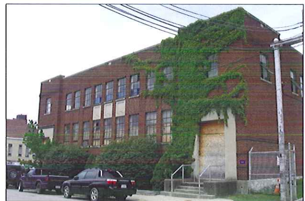
The State Road Commission Building prior to renovation.
