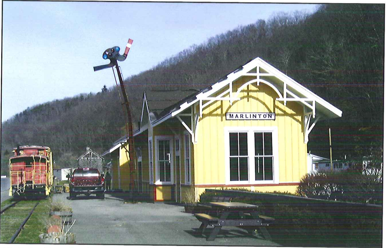
Marlinton Depot Project Marlinton, West Virginia
