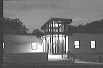
2009 Construction & Facilities Management Office Charleston, WV 2009 - Merit Award "Achievement in Architecture" AIA West Virginia Chapter
