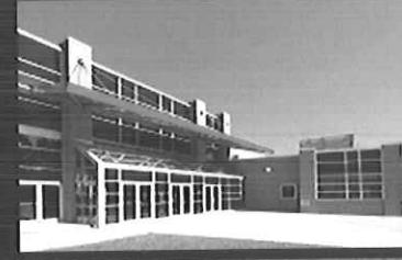
2004 St. Albans High School St. Albans, WV 2004 - Impact in Learning Award "Effective Transformation" Education Design Showcase "Outstanding Building Design" American School & University "Outstanding Building Design"
